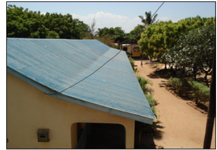
We also replaced the rusty roofs, which had become leaky. It is easy to appreciate the difference: on the left is the old roof, and on the right is the new one.
