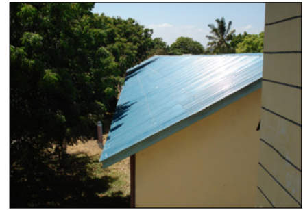
We also replaced the rusty roofs, which had become leaky. It is easy to appreciate the difference: on the left is the old roof, and on the right is the new one.
