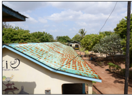
We also replaced the rusty roofs, which had become leaky. It is easy to appreciate the difference: on the left is the old roof, and on the right is the new one.
