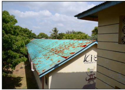
We also replaced the rusty roofs, which had become leaky. It is easy to appreciate the difference: on the left is the old roof, and on the right is the new one.
